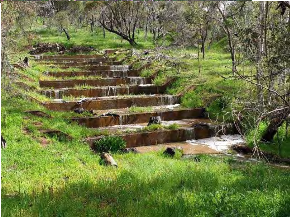
Top: Pelham Reserve, Duke Street Toodyay (2021-09-14) Bottom: Pelham Brook Spillway (2021-08-10)
